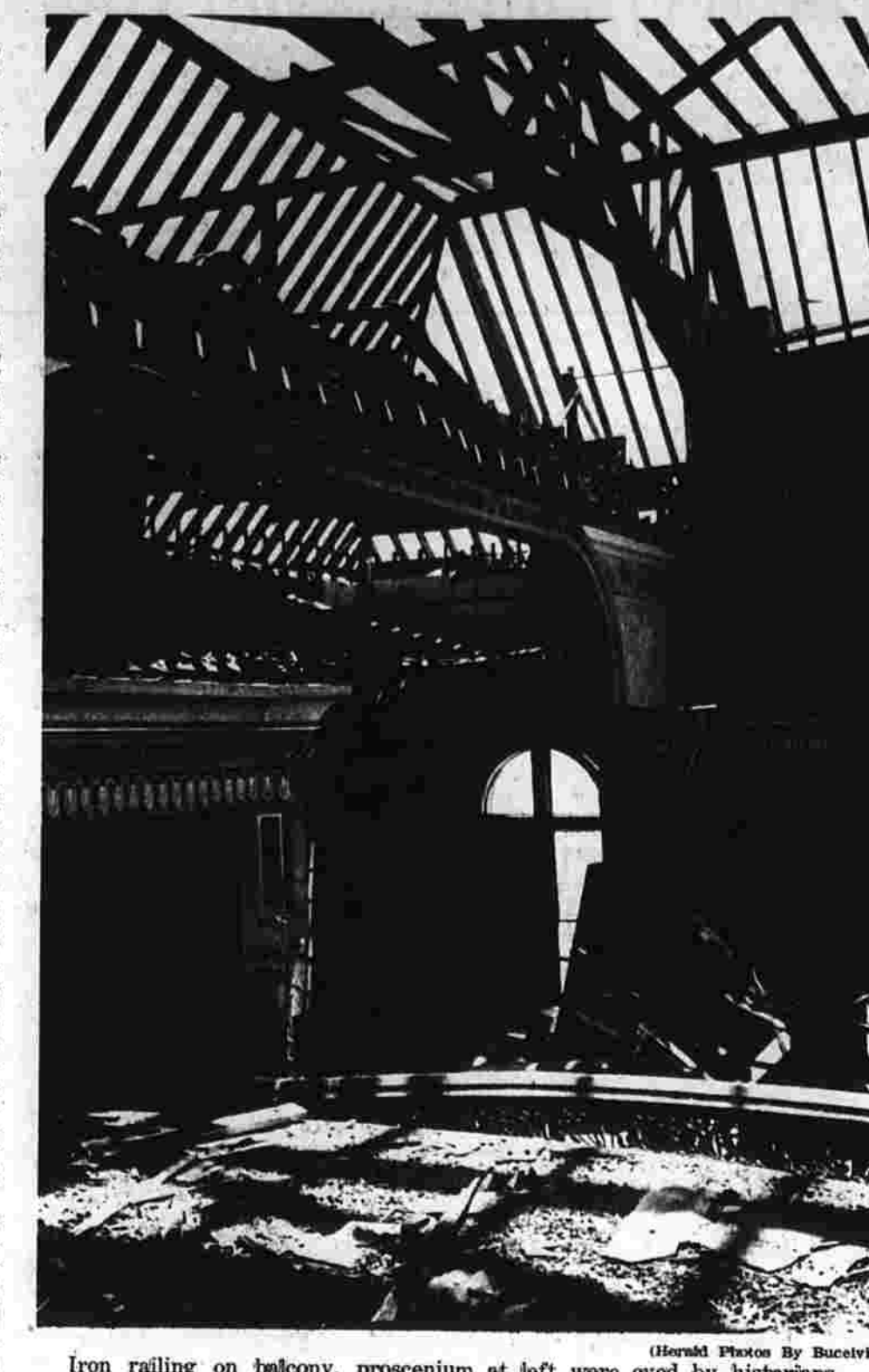
Iron railing on balcony, proscenium at left is eyed by historians.
